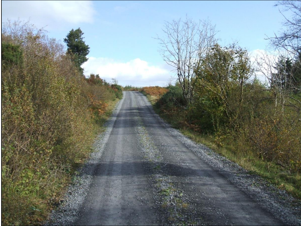
Photo 1 Example of an existing excavated access track on site
