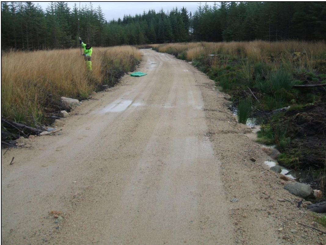
Photo 2 Example of an existing floating access track on site
